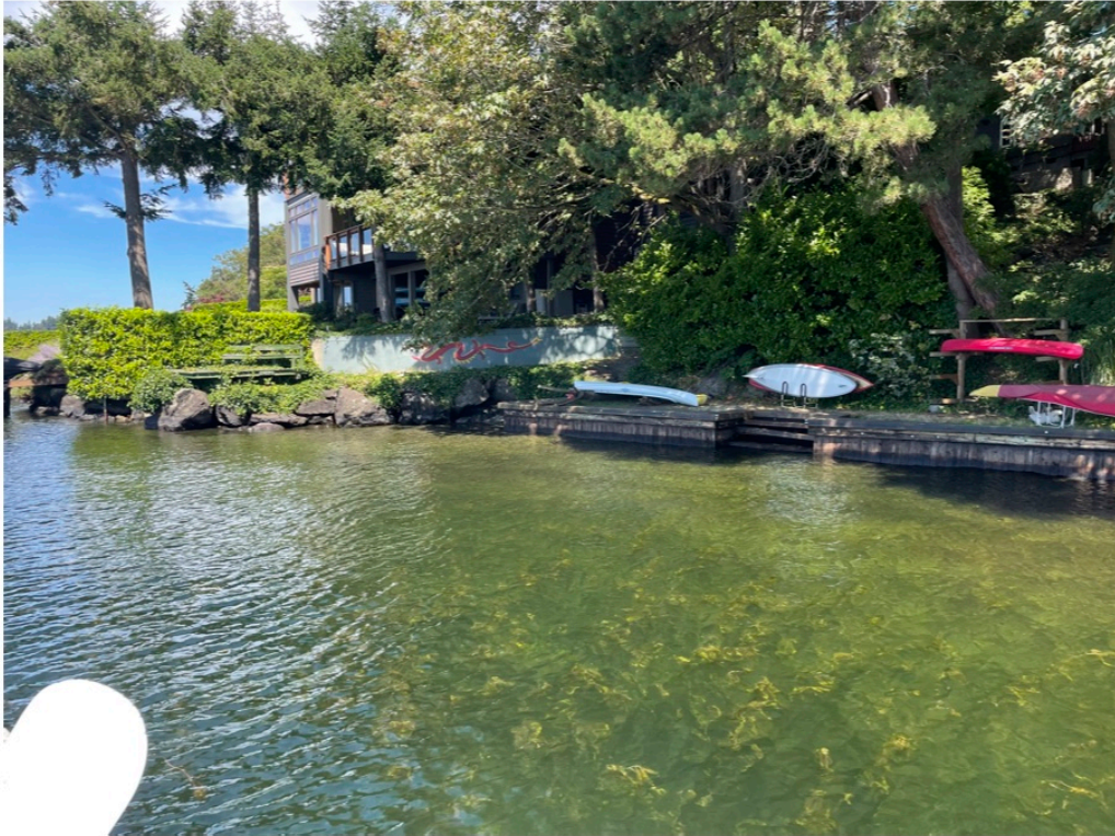
Photo 3 - Shoreline conditions looking north of the dock. Bulkhead to be replaced.
