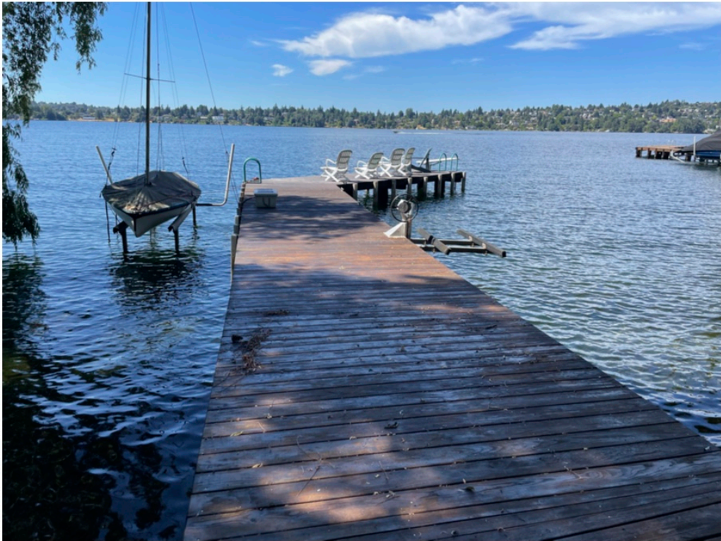
Photo 1 - Existing dock looking waterward.
